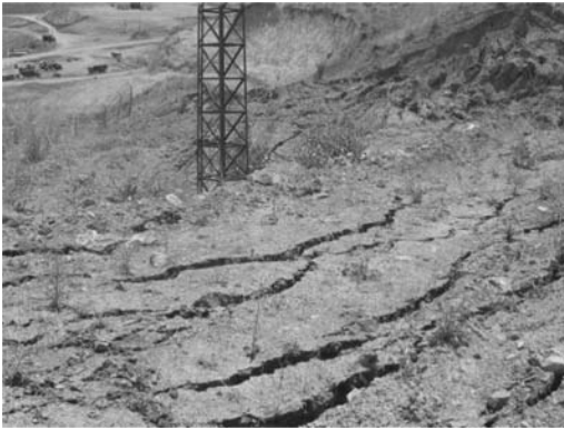
Figure 1. Tention cracks near borehole BH 55 due to slipping.
