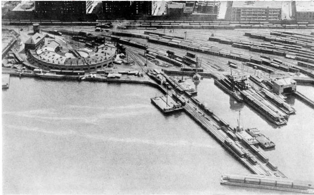
AN AÉRIAL VIEW OF THE WEST 72D STREET FREIGHT YARDS, NEW YORK, SHOWING A BIT OF RIVERSIDE DRIVE IN THE UPPER LEFT CORNER Below Riverside Drive is a roundhouse, "the iron horses' stable," where some twenty engines may be sheltered. In the lower right corner is a car ferry. The canteloupe loaded into a refrigerator car in Arizona requires about two pounds of coal to bring it to an Atlantic seaboard breakfast table, while a half-pound of ice and locomotive fuel is used in bringing an orange from the Imperial Valley orangery to the Boston market.
